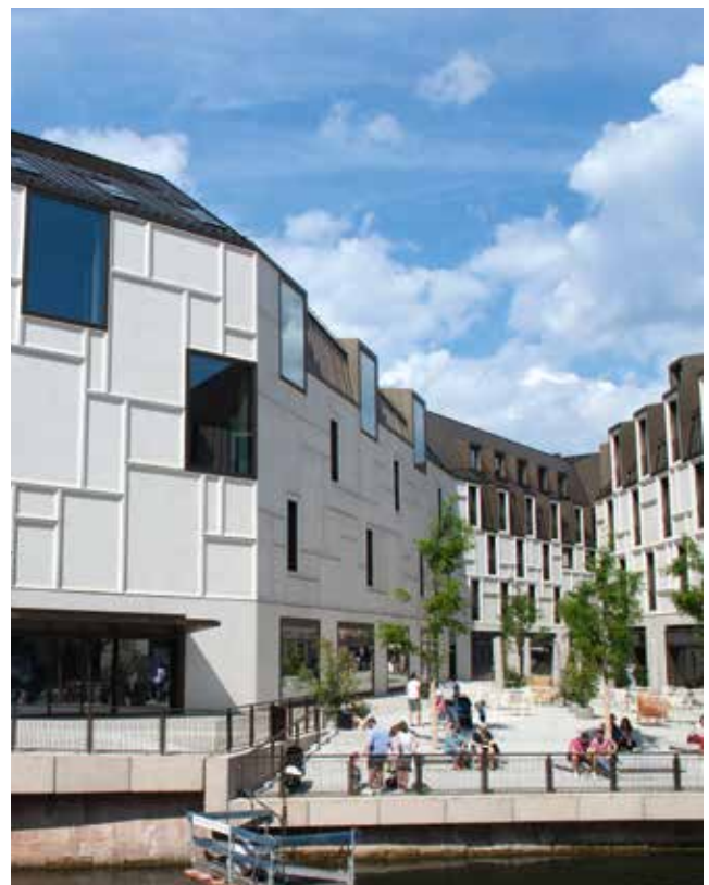
Augustinerhof in Nuremberg Since being opened in 2021, the Augustinerhof is home to the Deutsches Museum as well as hotels, shops and eateries. 950 luminaires and 11 central battery systems from the RP Group are used in the 23 000 m 2 complex.
